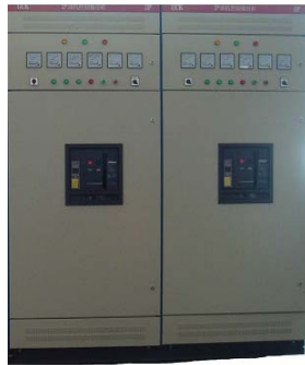
Paralleling/synchronizing System
