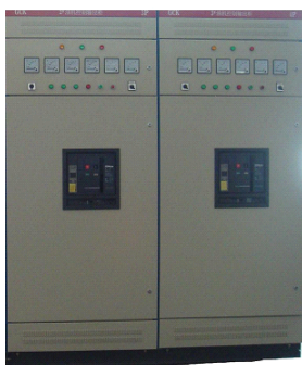
Paralleling/synchronizing System
