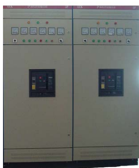
Paralleling/synchronizing System
